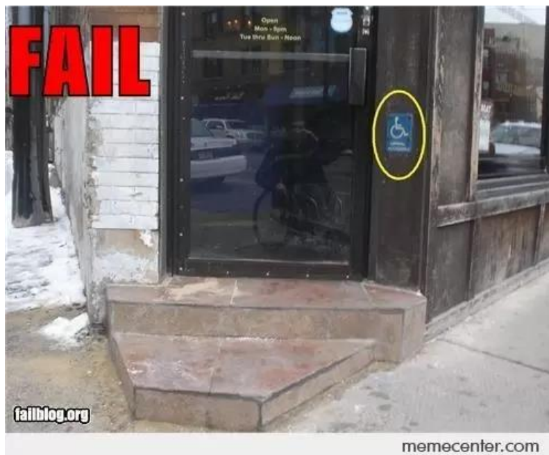
Figure 32: Accessibility fail (source: https://www.memecenter.com/fun/64537/Wheelchair-AccessibilityFAIL ).
